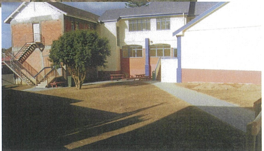
Right: The view from the tennis court side when 'Original High School Building' was demolished in 1999
